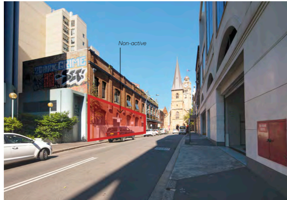
Above: Valentine Street Current Condition, Google Images
